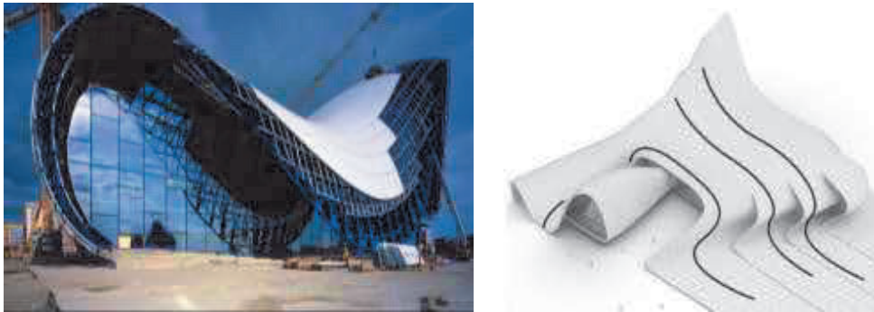
Figure 13. H. Aliyev Center, Space Frame and Boot Column Examples.
